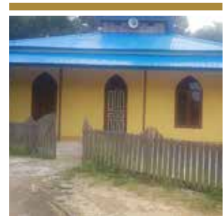
Renovasi Mushola Musalla Renovation
