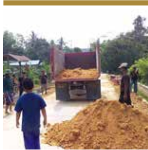
Pengurukan Bahu Jalan Road Shoulder Backfilling
