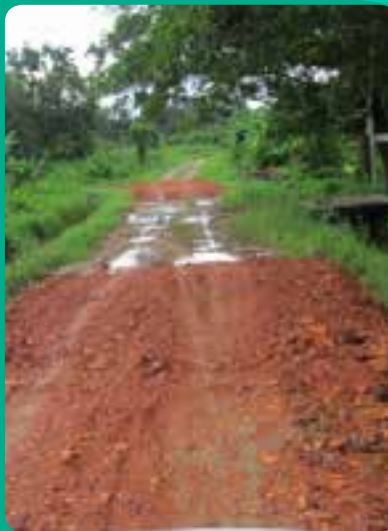
Bantuan Material Laterit Pengerasan Jalan Nanas RT 11 Laterite material aid for Nanas Road RT 11 street paving
