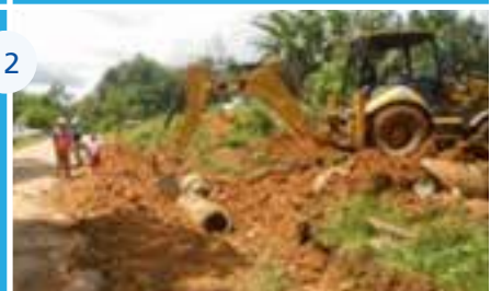
Pemasangan gorong-gorong di jalan masuk SDN 06 Bingin Teluk. Installation of sewer system at the entrance of SDN 06 Bingin Teluk.
